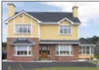
Casement Georgian with uPVC with hardwood front door unit
